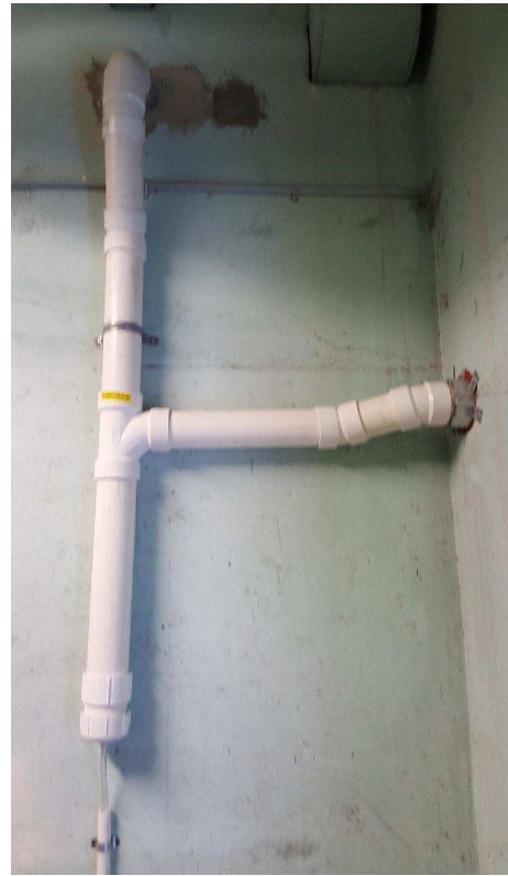
Vent piping coming through the foundation wall from the corridor drop ceiling and into the receiving room.
