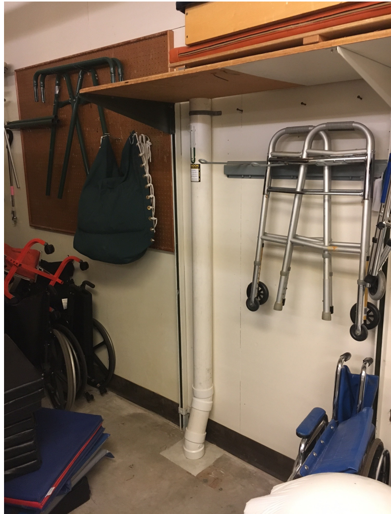
Suction point location in a storage coral of the wood shop.
