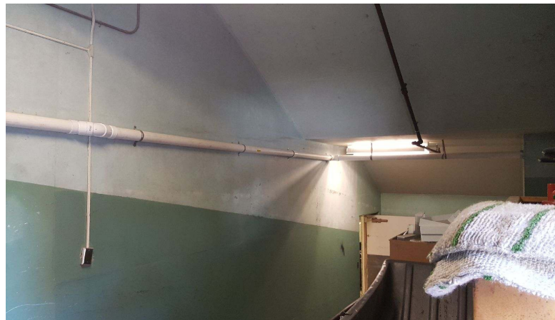
Vent routing from the receiving room through the receiving corridor and to the exterior foundation wall.
