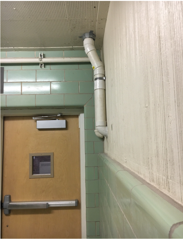
Vent routing from Faculty Serving room up into the drop ceiling of the corridor.
