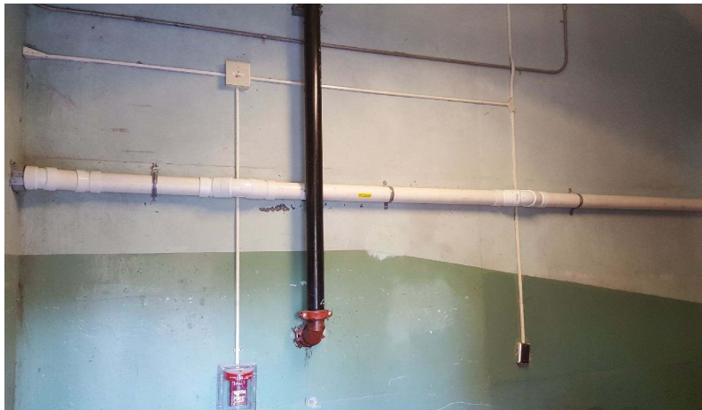
Vent routing from the receiving room through the receiving corridor and to the exterior foundation wall.
