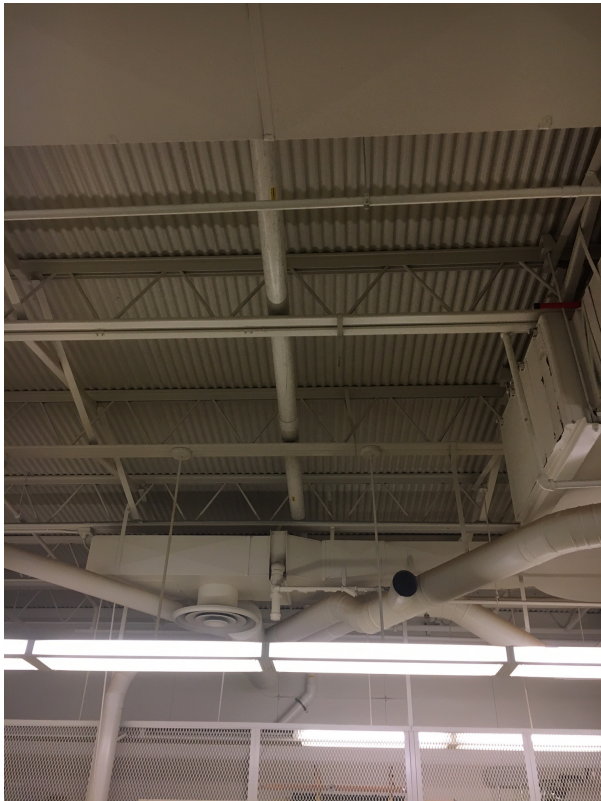
This portion of system #1 is the vent piping continuing from the suction point across the wood shop and through the roof deck to the mitigation fan on the roof.
